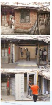
and bathrooms; installation takes only one day, so the residents don't need to move out during the upgrade. Each panel can be connected with a simple Allen wrench (a tool commonly used to assemble Ikea furniture). Residents also can choose to connect their graywater plumbing lines to a septic tank in the courtyard and install a composting toilet.
